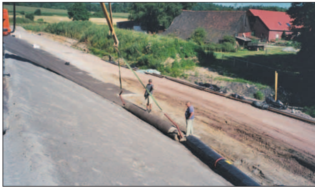
The diagram shows the construction of the embankment area at Rotbach. The recognisable yellow GCL, NaBento® RL-N, protects the underlying coal spoil tailings material.
